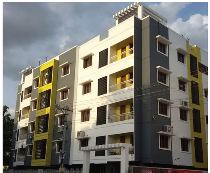
SAI CHARAN, Sathya Sai Nagar, Madurai
